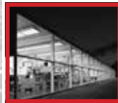
The Republic - Newspaper Plant & Offices Columbus, Indiana
