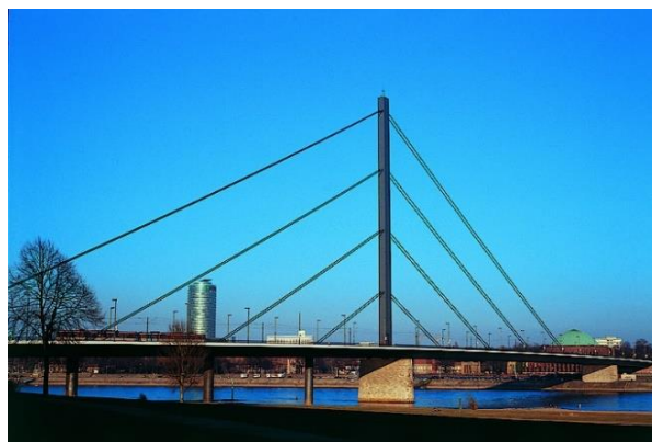
Figura 2.25 – Oberkassel Bridge, Alemanha. (DUESSELDORF-TOURISMUS, s.d)
