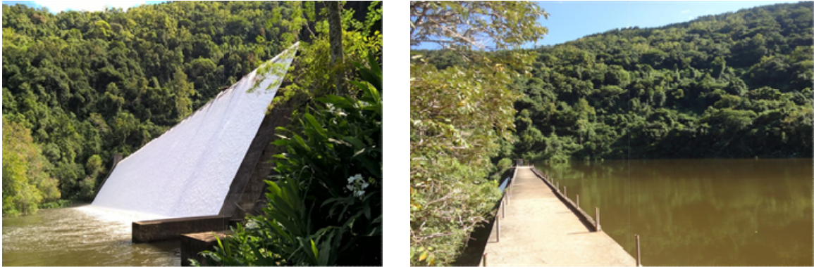
Figure 7.1: a) Lateral view of the spillway, on the left; b) water surface near the dam, on the right.
