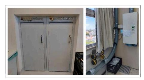
Fig. 3. Left: elevator that connects the main hospital warehouse to the ICU pharmacy; right: pneumatic tube and capsules for placing materials.
