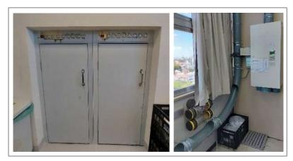
Figure 13 - Left: elevator that connects the main hospital warehouse to the ICU pharmacy; right: pneumatic tube and capsules for placing materials.
