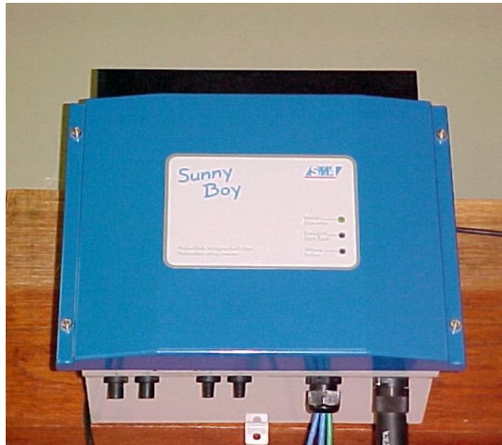
Figura 4.2 Inversor CC/CA modelo Sunny Boy 1100E.
