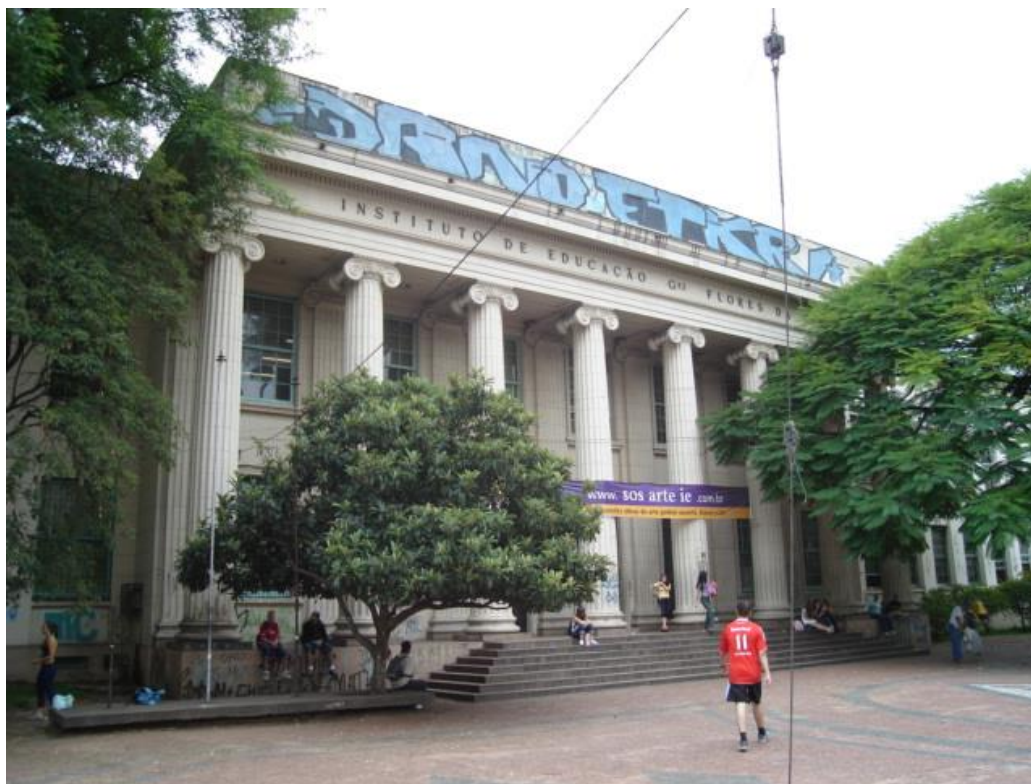
Figura 3 – Fachada principal IE
