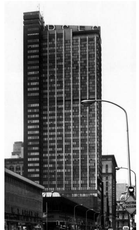
Fig. 236: George Howe e William Lescaze, Philadelphia Savings Fund Society (PSFS) Building, Filadélfia, Pensilvânia, 1929-1932.-1930.
