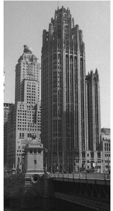
Fig. 115: Raymond Hood e John Mead Howells. Torre do Chicago Tribune, vencedora do concurso. Chicago, Illinois, 1923-1925.
